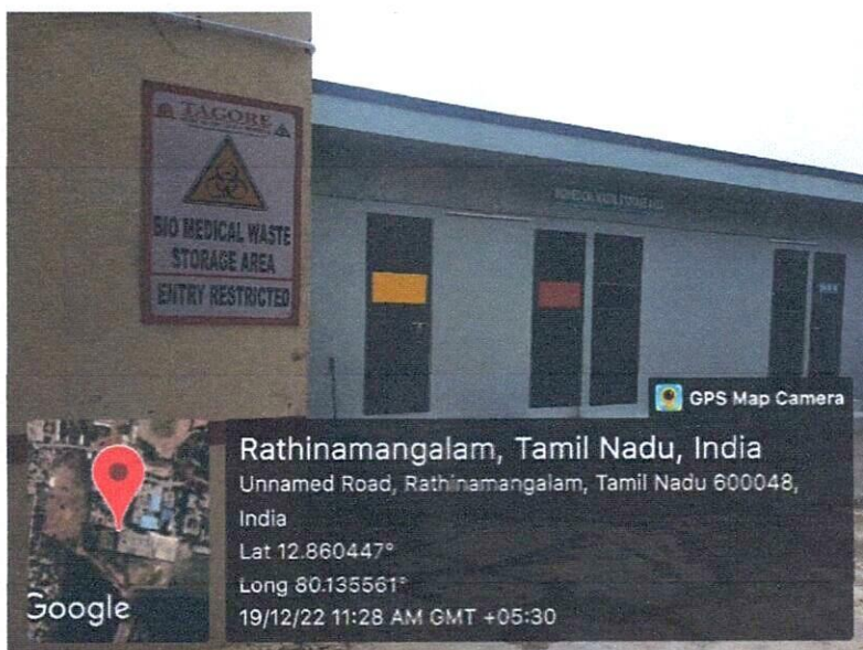
Biomedical Waste management area
